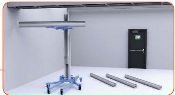
Use the material lift to raise the wall panel
