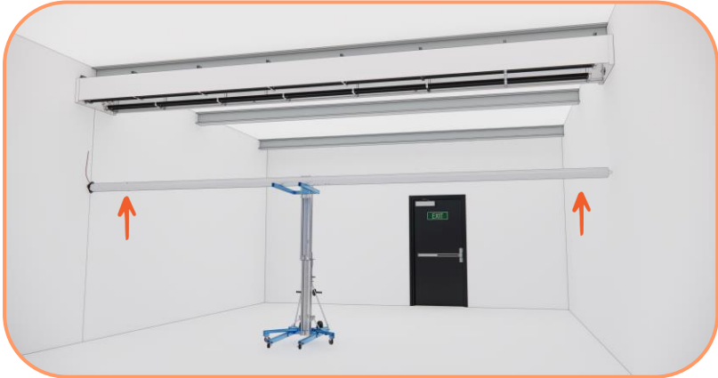
Use the material lift to raise the connected tubes to the housing system
