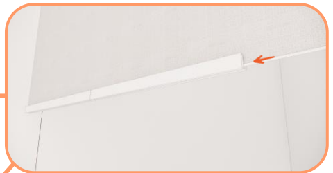
Slide in second weight bar and prepare to stretch the wall panel
