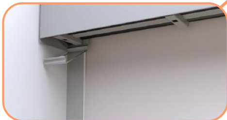
Insert the beginning under-housing access panel
