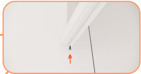
Insert the first screw at the beginning of the weight bar
