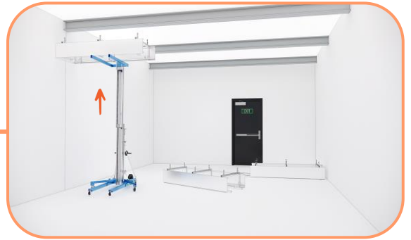
Use the material lift to raise the first housing unit
